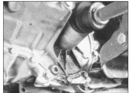
Gearbox oil can leak from the seals at the inboard ends of the driveshafts.
