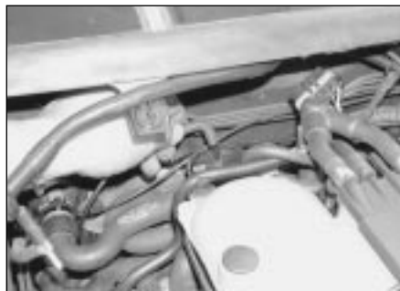
4.29b . . . then disconnect the vacuum hose from the heater cut-off valve
