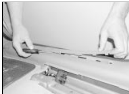
28.5a Prise the cover strip from the sill trim panel
