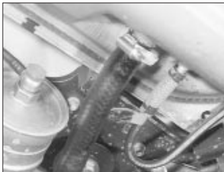
5.7 Fuel tank supply (left) and return hoses
