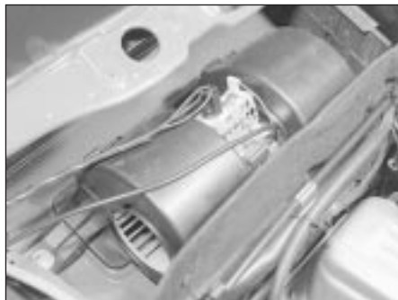
29.5 Blower motor showing wiring connections
