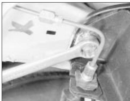
10.35 Unscrewing crossmember side bracket mounting bolts
