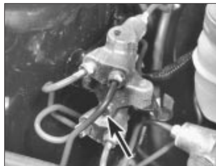
14.2 In the event of failure, fluid will seep from pressure regulating valve plug (arrowed)
