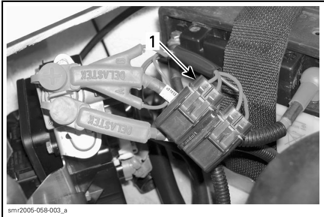
1. Charging system fuse
