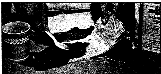
Fig. 76—Applying Resin Mixture to Fiber Glass
