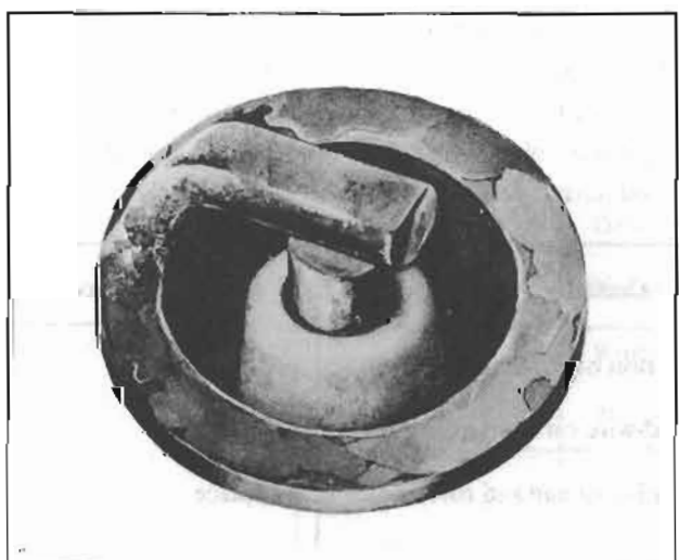
Fig. EE-97 Overheating (I)
